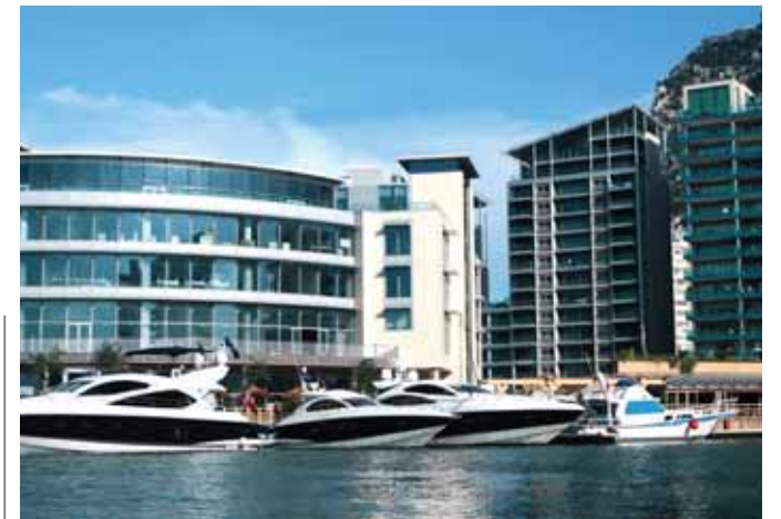
Award-winning Royal Ocean Plaza (right) in the making with the Casino on distinctive Leisure Island (left) opening in January.
