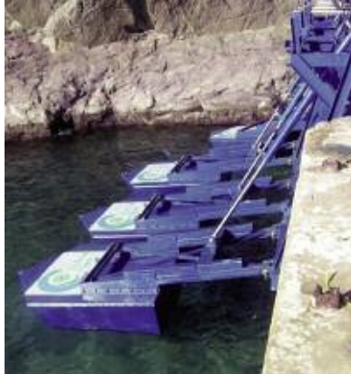
Floaters produce power from waves at EWP pilot installation
